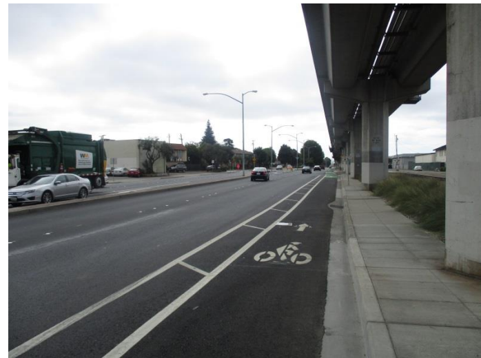
VIEW LOOKING SOUTH SHOWING NEW BIKE LANE
