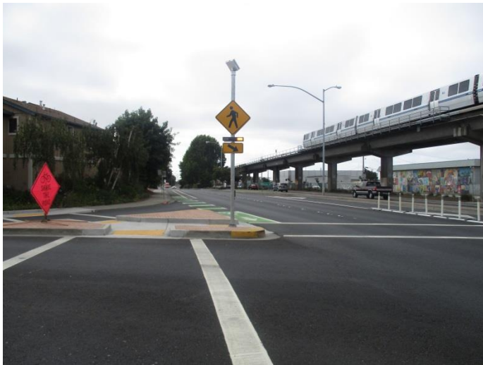
VIEW LOOKING SOUTH FROM CASTRO STREET INTERSECTION (WITH NEW FLASHING BEACON)
